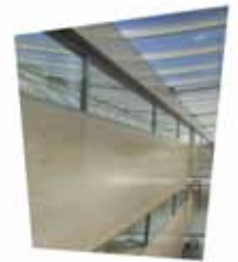
mirror-panel (polycarbonate) sticked with alumi- um-coupond-panel
